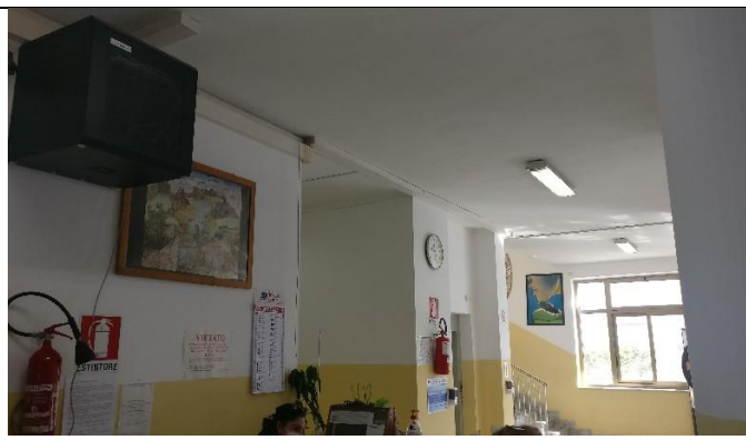
Figure 6-14 Armadio e Switch rete Wifi piano terra
